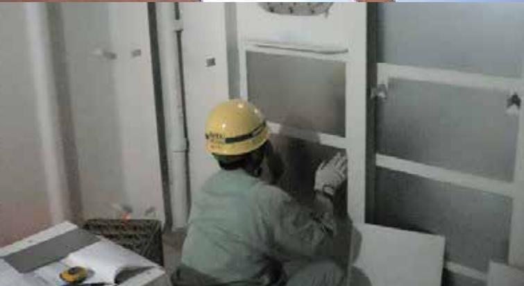
Application of Calmmoon Marine with Spot Welding
